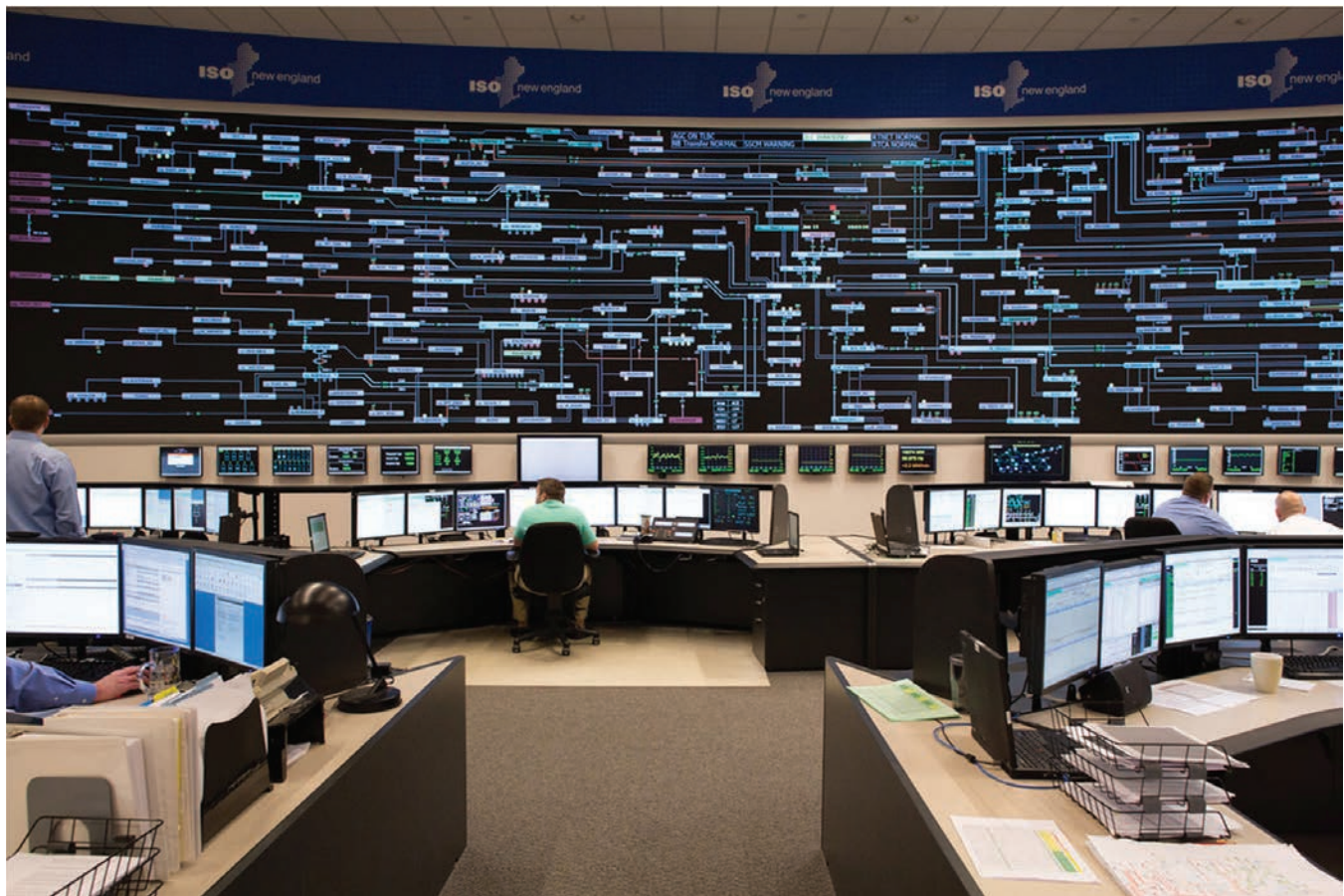
FIGURE 4.7 ISO New England control room. SOURCE: ISONE (2013).
