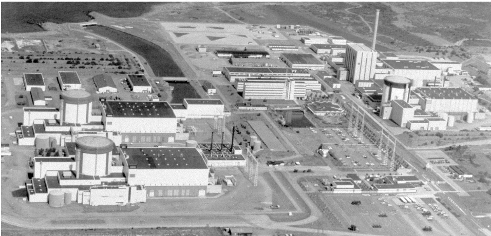
Figure 19.2 Main components of a pressurized light water cooled and -moderated nuclear power reactor (PWR) and a view of the Ringhals plant (Sweden) with 3 PWRs and 1 BWR.
