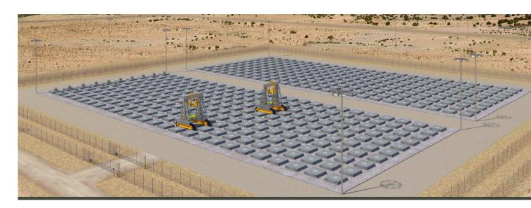
Figure 2.6: 500 cask Hi-Store pad. Hi-Store uses a vertical, below ground cask.
