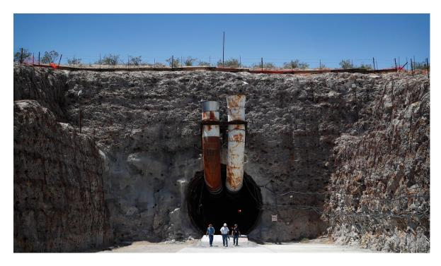
Figure 8.1: Rust in the middle of the Nevada desert. Nuclear quality Yucca Mt. ventilation ducts
