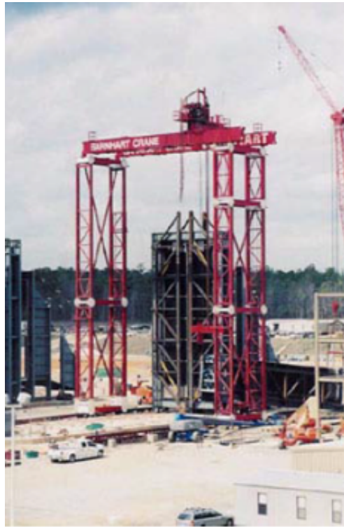
Figure 1-11. A lift tower [17] of similar size to that needed for Mk1 construction, being used to assemble a heat recovery steam generator.
