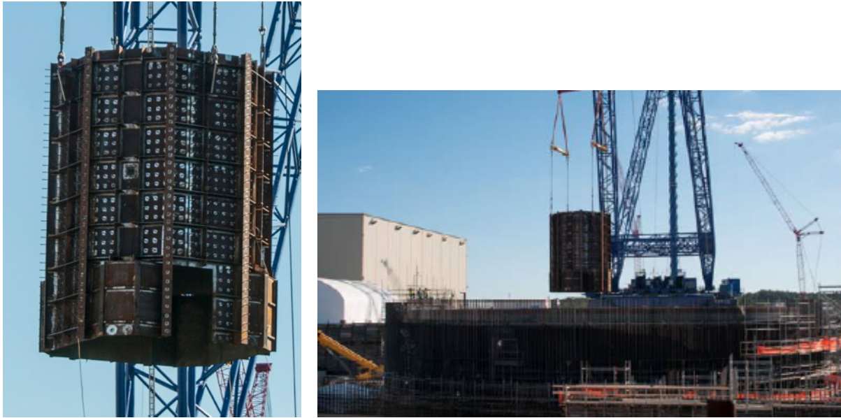
Figure 1-9 V.C. Summer Unit 2 AP1000 Reactor Cavity Module CA04 being installed Sept. 27, 2013 [14].
