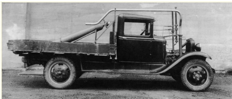
Figure 45 Norsk Hydro's ammonia-fueled truck circa 1933
