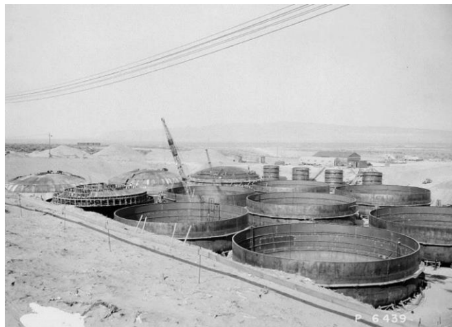
Figure 82 Hanford’s waste tanks during construction (typically 1 million gallons each)
