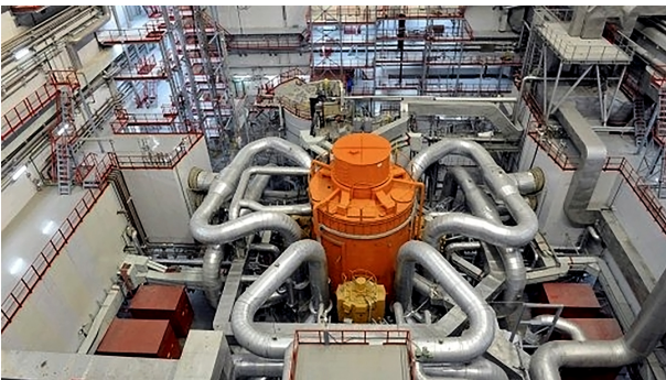
Figure 1. Photograph of the Russian BN-800 in operation since 2016.
