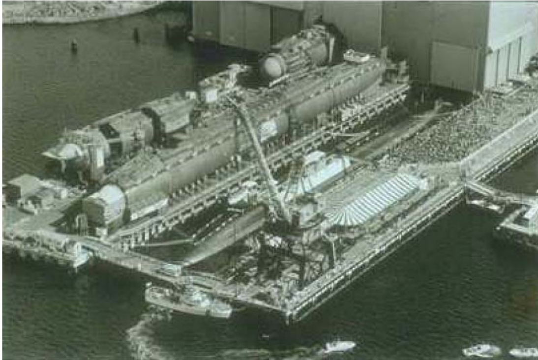
Figure 45: Christening of a Trident Submarine, with Two Other Submarines in Different Stages of Assembly
