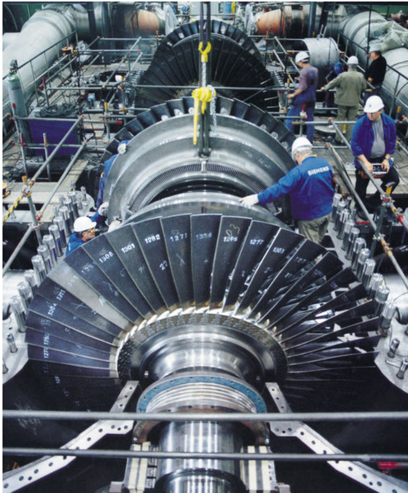
Figure 14: A Siemens Steam Turbine with Open Case
