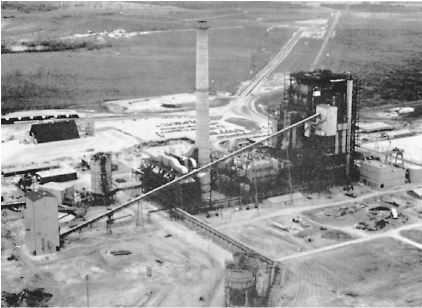
Figure 12.2 San Miguel Power Project. ( Babcock & Wilcox, a McDermott company. )
