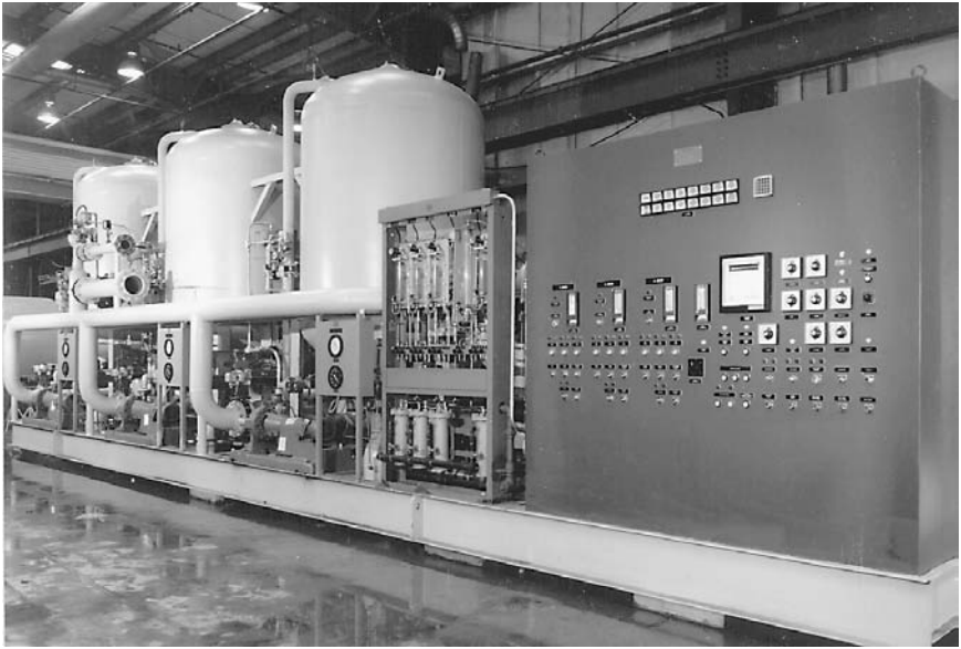
Figure 11.14 Condensate polisher, skid-mounted Powdex system. ( The Graver Company, Graver Water Division. )
