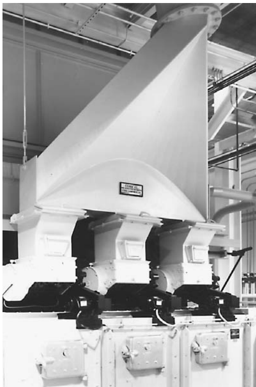
Figure 5.9 Conical nonsegregating coal distributor across stoker inlet. ( Stock Equipment Company. )
