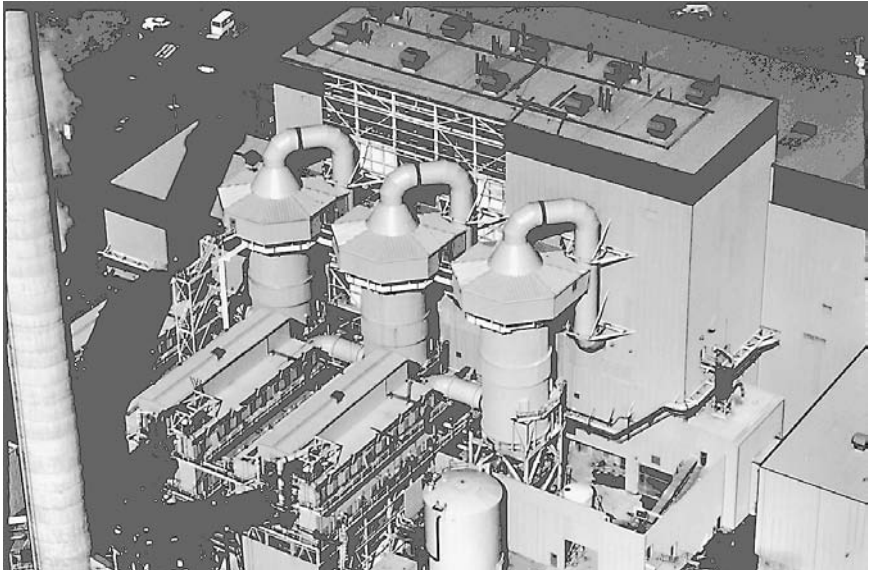
Figure 12.26 Vertical dual fluid spray-dryer scrubbers and fabric filters for control of emissions from three MSW-fired boilers at a 2250-ton/day waste-to-energy plant. ( Wheelabrator Air Pollution Control, Inc. )
