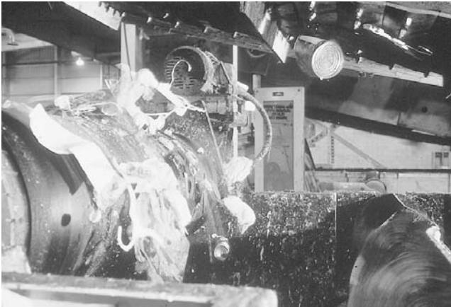
Figure 13.22 Magnetic separator for recovery of ferrous materials. (National Ecology, a Babcock & Wilcox company.)
