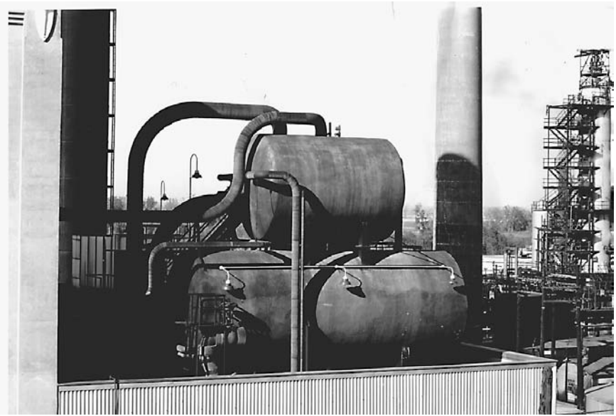
Figure 11.6 Deaerator outside location on roof of boiler building. ( The Graver Company, Graver Water Division. )
