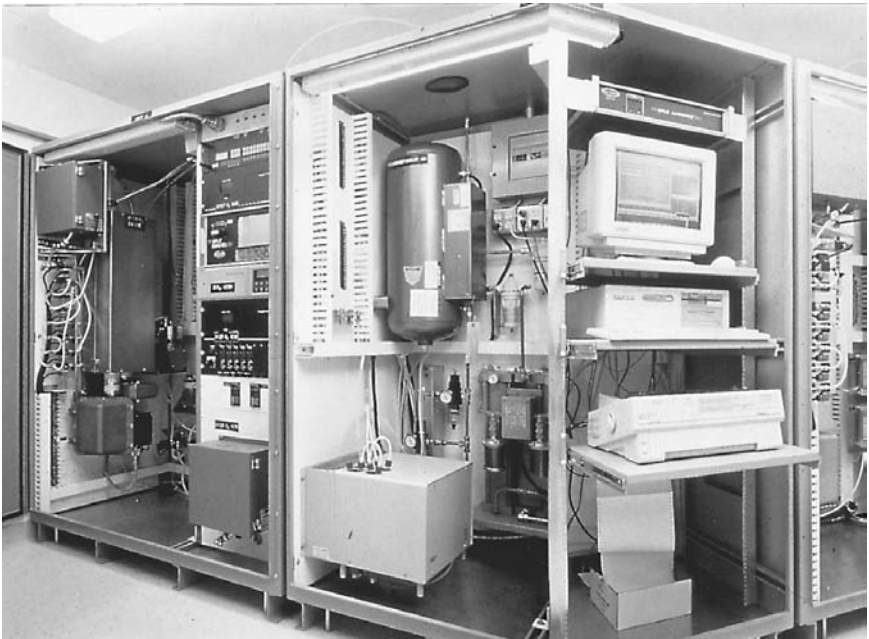
Figure 6.40 Continuous-emission-monitoring (CEM) system.
