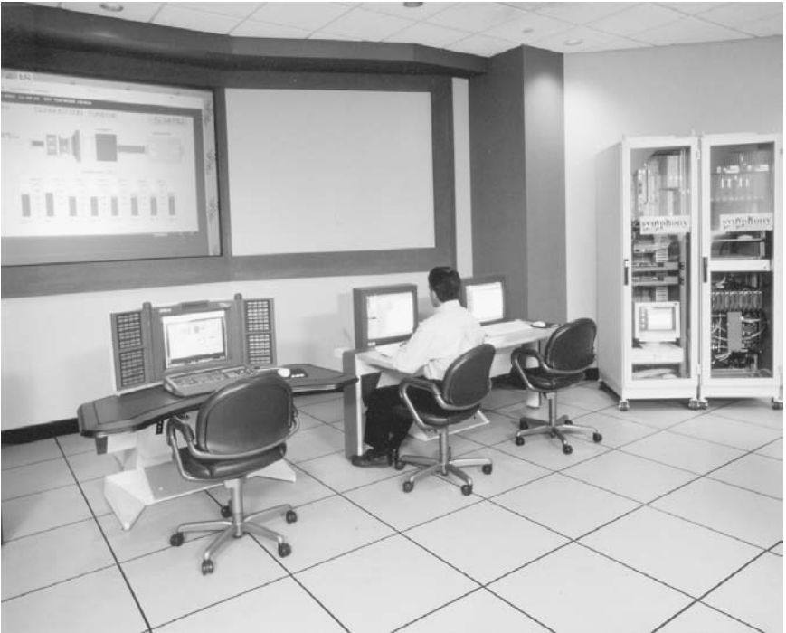
Figure 6.41 ABB SYMPHONY control system with overhead display. (ABB, Inc.)
