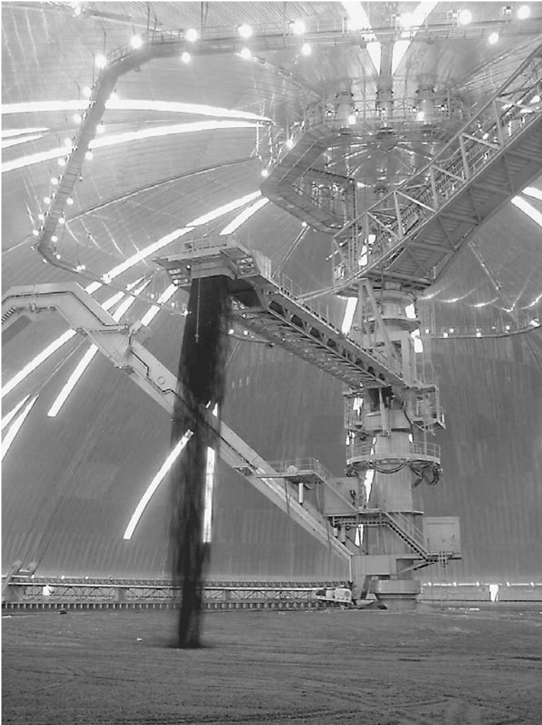
Figure 4.13 Coal conveyor system in operation ( Geometrica, Inc. )
