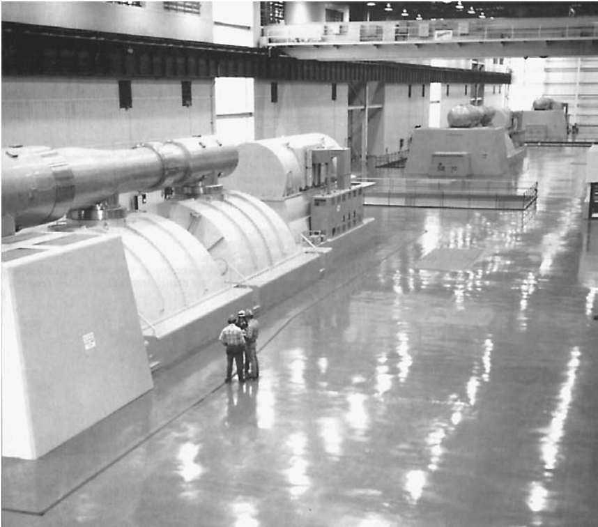
Figure 9.5 Turbine room of utility power plant showing three 600-MW steam turbine generators. ( Babcock & Wilcox, a McDermott company. )
