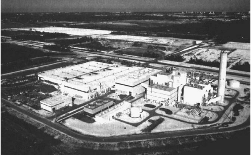
Figure 13.14 Aerial view of a 2000-ton/day RDF waste-to-energy plant, Palm Beach County, Florida. ( Babcock & Wilcox, a McDermott company. )
