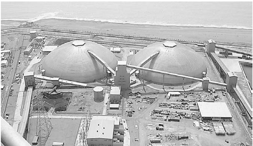
Figure 4.11 Coal storage domes for power plant in Taiwan. ( Geometrica, Inc. )
