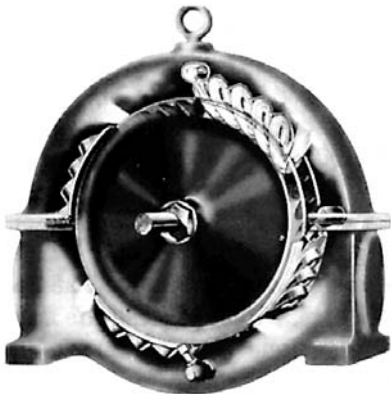
Figure 9.3 Action of steam in a small turbine.
