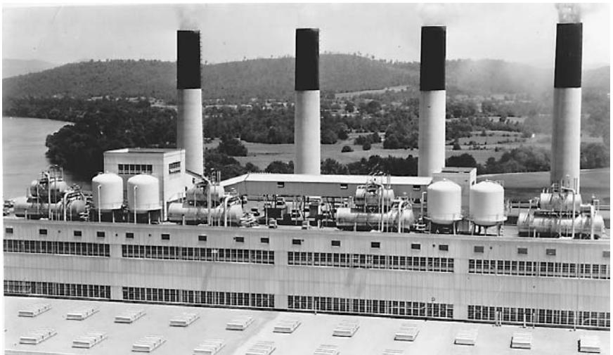
Figure 11.7 Series of deaerators located on roof of boiler building for large utility plant. ( The Graver Company, Graver Water Division. )
