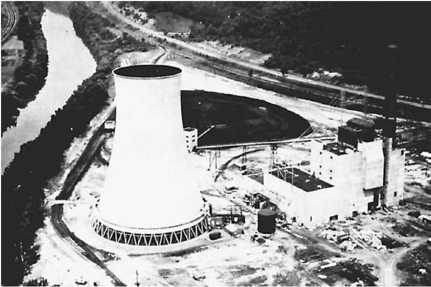
Figure 9.53 Hyperbolic natural-draft cooling tower. (Marley Cooling Technologies.)
