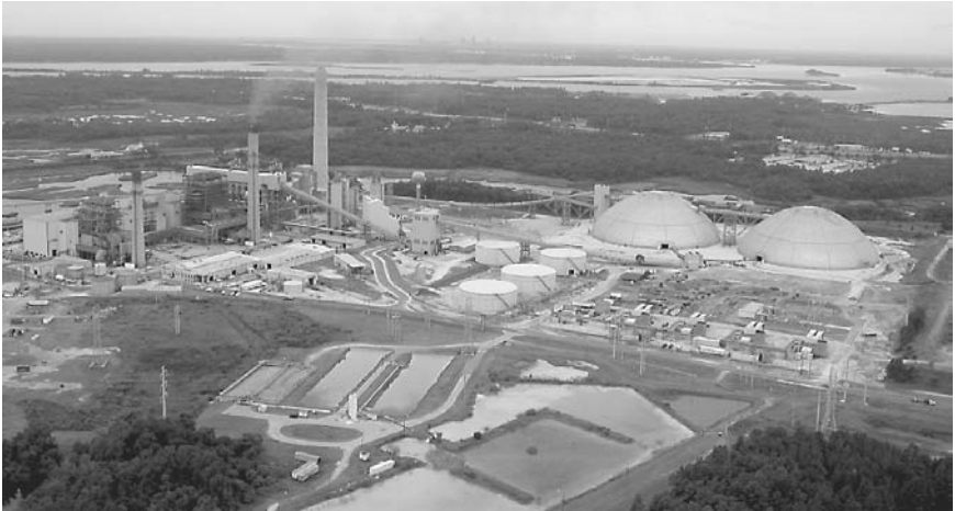
Figure 1.6 Large-scale circulating fluidized bed (CFB) combustion project with coal storage domes. (Photo courtesy of JEA.)
