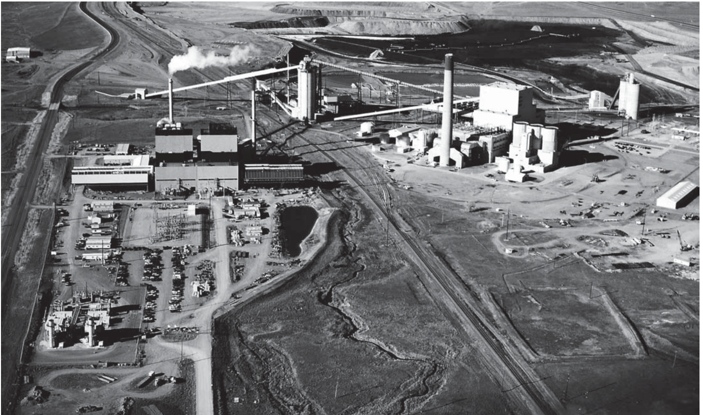
Fig. 27 This energy complex in the northern U.S. includes four coal-fired steam systems, ranging from 80 to 330 MW, installed over a 25-year period.
