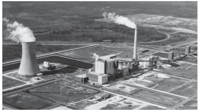
Fig. 9 Coal-fired utility power plant.
