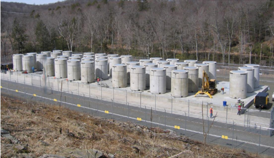
Figure 2.2: Connecticut Yankee Dry Cask Storage Facility. If CT Yankee had been a coal plant and we tried to store the coal waste on the same pad, it would be a column 7000 feet high.
