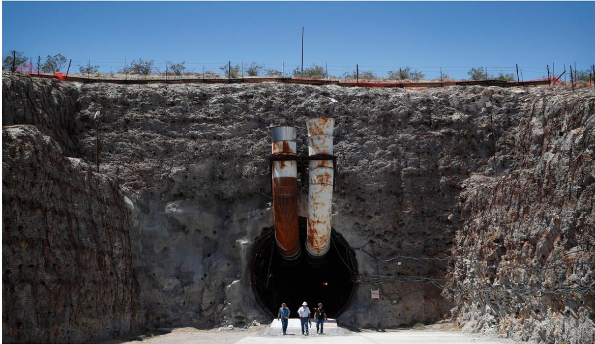
Figure 8.1: Rust in the middle of the Nevada desert. Nuclear quality Yucca Mt. ventilation ducts
