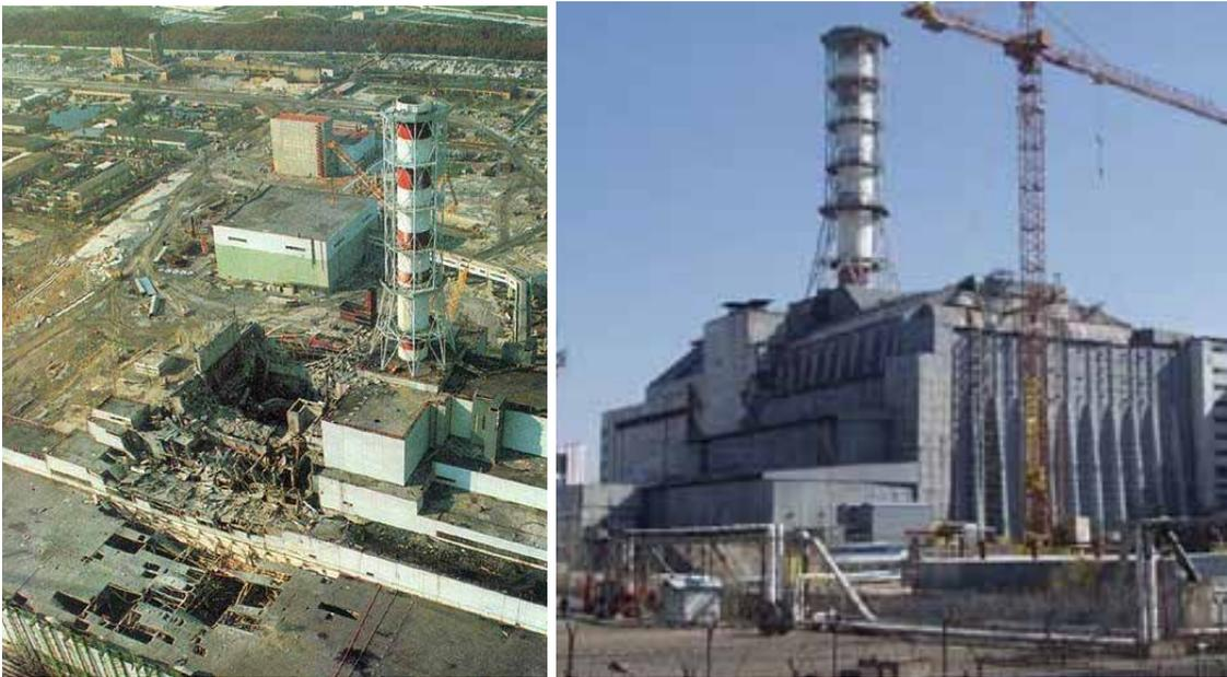
Figure 4.10: Left: Chernobyl Unit 4. Unit 3 is on the right. Right: Sarcophagus in place.
