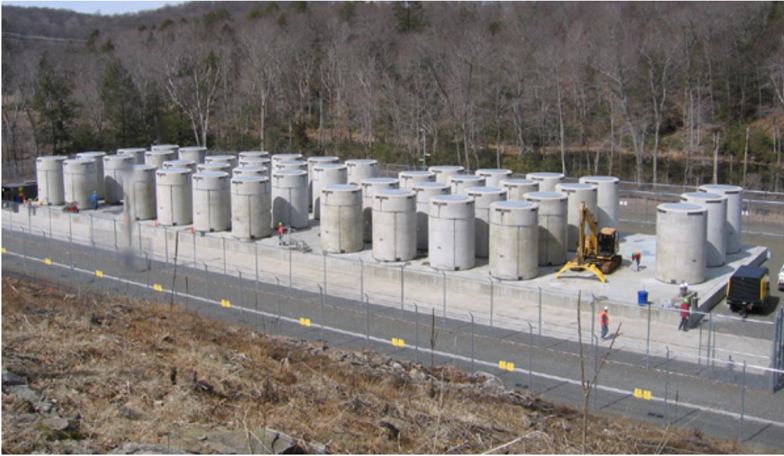
Figure 1: Connecticut Yankee Dry Cask Storage Facility. If CT Yankee had been a coal plant and we tried to store the coal waste on the same pad, it would be a column 7000 feet high.
